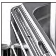
Condensate return system
